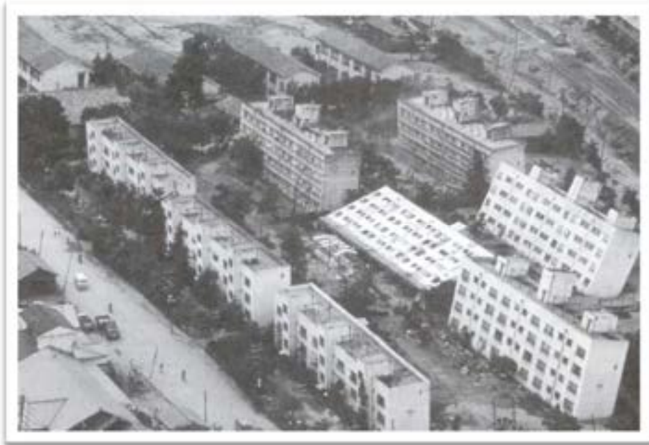
Fig. 3.19. Soil liquefaction under the foundation due to the earthquake and collapse of some structures, Niigata, Japan 16 th of June 1964, 7,6 Richter
