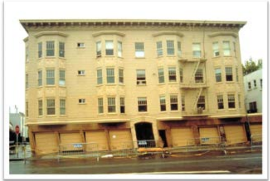
Fig. 3.6. Civil building with weak garage base floor, San Francisco, California, Loma Prieta earthquake, 17 th of oct 1989, 6,9 Richter, National Information Service for Earthquake Engineering (NISEE), University of California, Berkeley
