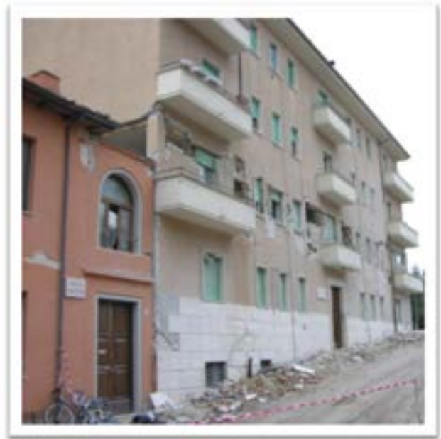
Fig. 3.14. Damage to the four-storied building due to pounding to the two-storied nearby building, L'Aquila earthquake, Italy, 6 th of April 2009, 5,8 Richter
