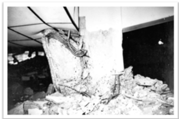
Fig. 3.5. Damage due to general torsion of the building, column damage and falling of upper floor to the right due to torsion, Hotel Terminal, Guatemala, 4 th of feb 1976, 7,5 Richter, USGS, Figure 74, Professional paper 1002, public image
