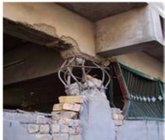
Fig. 3.10. Short columns, Algeria, 2003 (left), Failure of column due to partial masonry (right)
