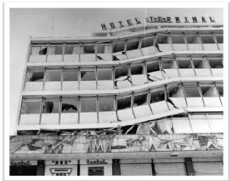
Fig. 3.4. Damage due to torsion with second level collapse, Hotel Terminal, Guatemala, 4 th of feb 1976, 7,5 Richter, USGS, Figure 55, Professional paper 1002, public image
