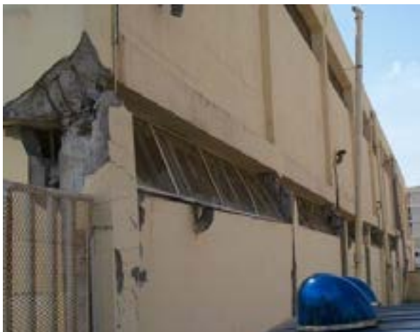
Fig. 3.10. Short columns, Algeria, 2003 (left), Failure of column due to partial masonry (right)
